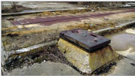
(above) Elevator doors and entranceway to magazine below at abandoned Nike launch site, Northampton Recreation center, Richboro.
