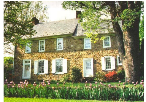
Bennet house in Richboro, believed to have been built about 1744 by William Bennet.
