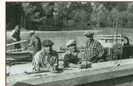
Circa 1942 photograph of workmen during the construction of the Churchville Reservoir Dam. Source: Courtesy of the Churchville Nature Center .
